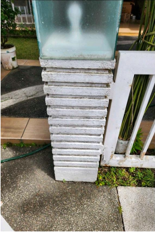
Existing light post - 5 sets
