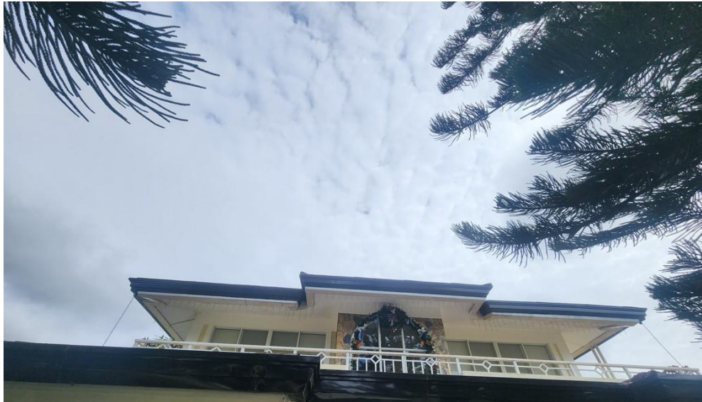
Front Roof Gutter (0.6mm) – 46.37 l.m
