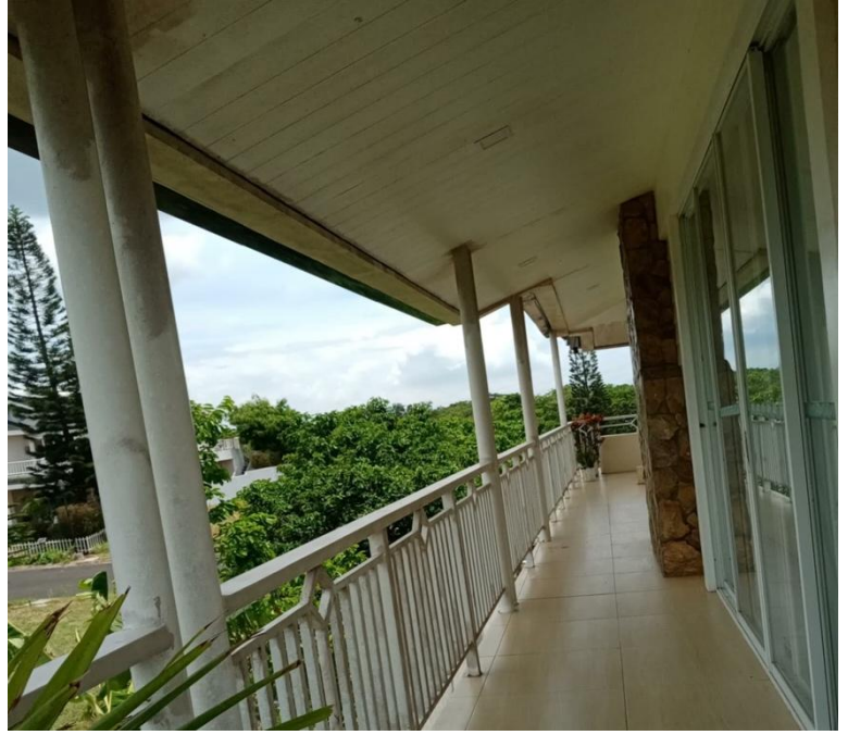
Existing roof eaves- 55 sq.m
