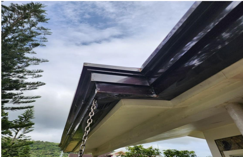
Existing gutter and downspout with chain
